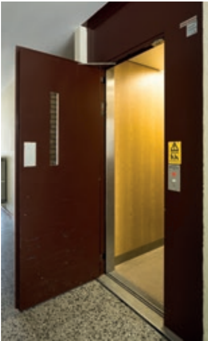
Old elevator before modernization.
